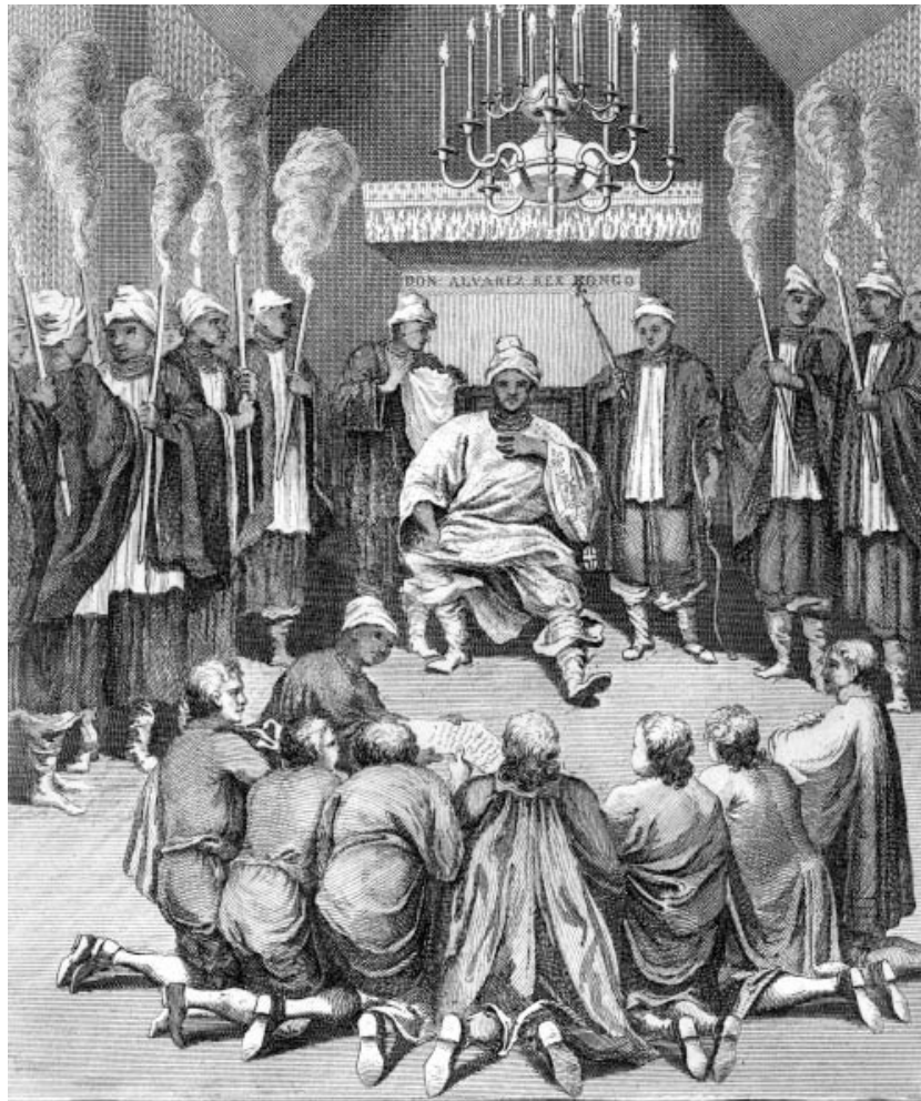
© Mary Evans Picture Library/The Image Works
