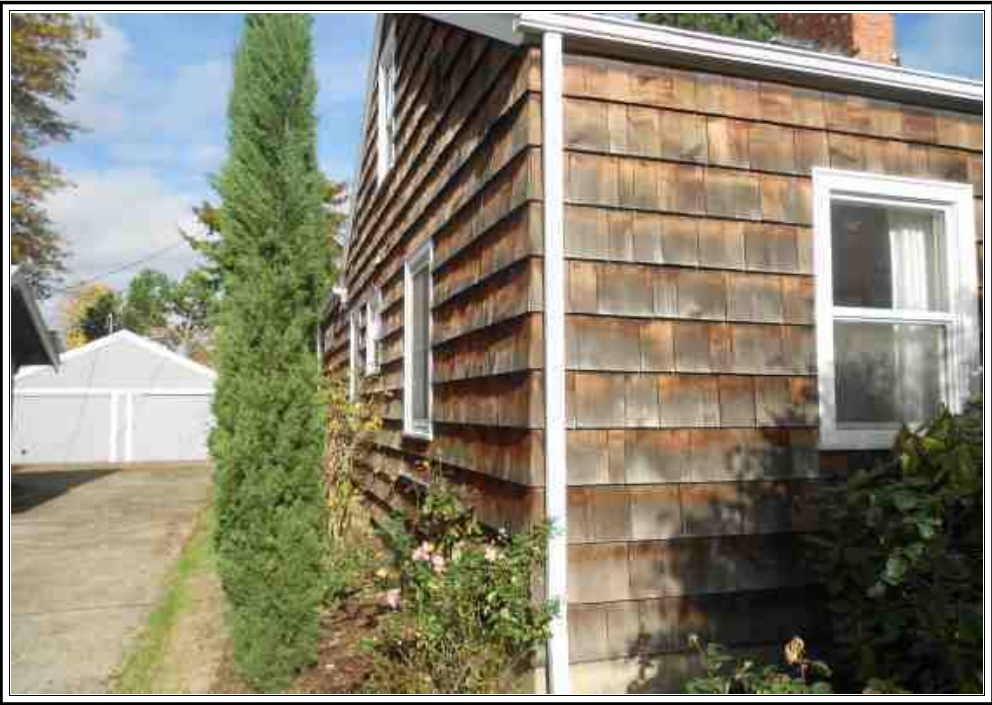
West Side of Subject
