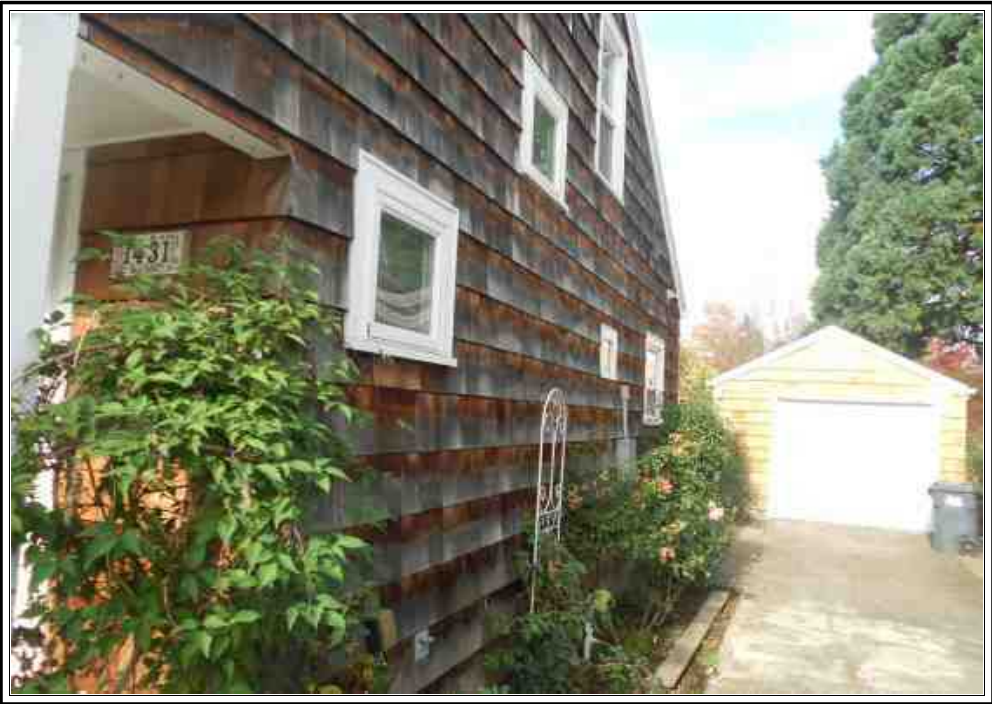
East Side of Subject
