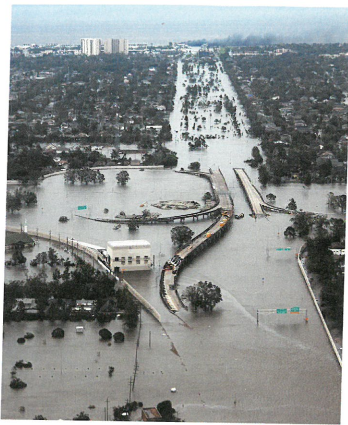
Figure 1.13 Post-Katrina New Orleans. The dams and levees built along the Mississippi River as it enters the Gulf of Mexico were unable to stop the flooding waters of Hurricane Katrina from inundating many portions of the city. (U.S. Coast Guard/Getty Images.)
