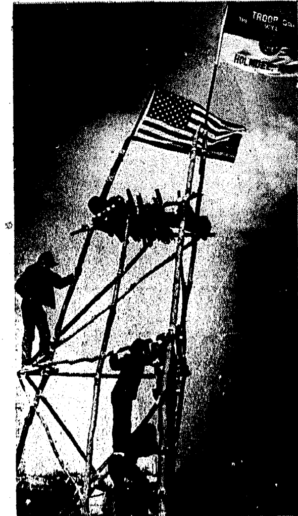
PIONEERING — Scouts from Troop 531, Holmdel, climb a wooden tower they constructed at Wolf Hill Farm, Oceanport. Project was part of Camporee in which some 3,000 Monmouth County Boy Scouts took part Saturday.
