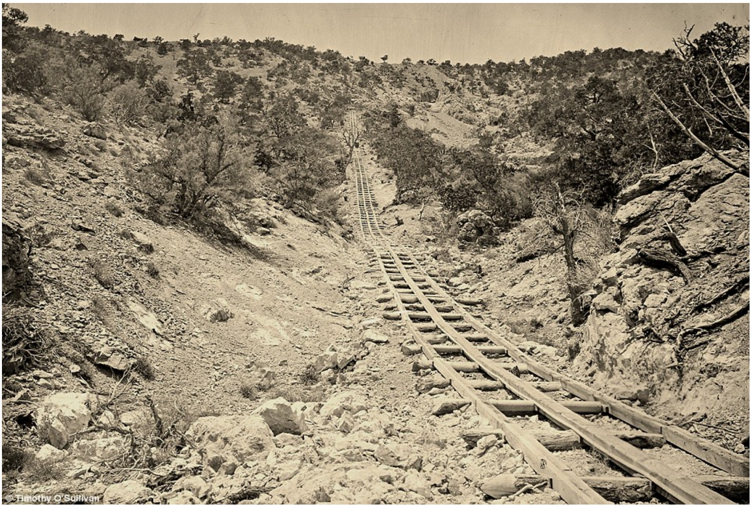
Early rails: A wooden balanced incline used for gold mining, at the Illinois Mine in the Pahranaagat Mining District, Nevada in 1871. An ore car would ride on parallel tracks connected to a pulley wheel at the top of tracks. Because of his work in U.S Civil War of 1861 to 1865, the organisers of the two geological surveys that he photographed knew that O'Sullivan was made of stern stuff and therefore could cope with the rigors of life outdoors far from home
